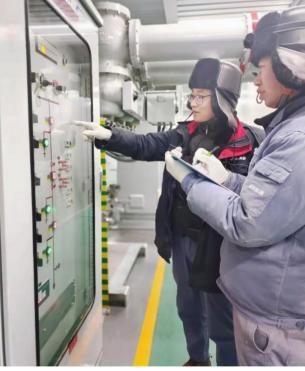
The on-duty personnel of Shangyi wind farm inspects the 220kV main transformer and switch cabinet in severe cold weather
